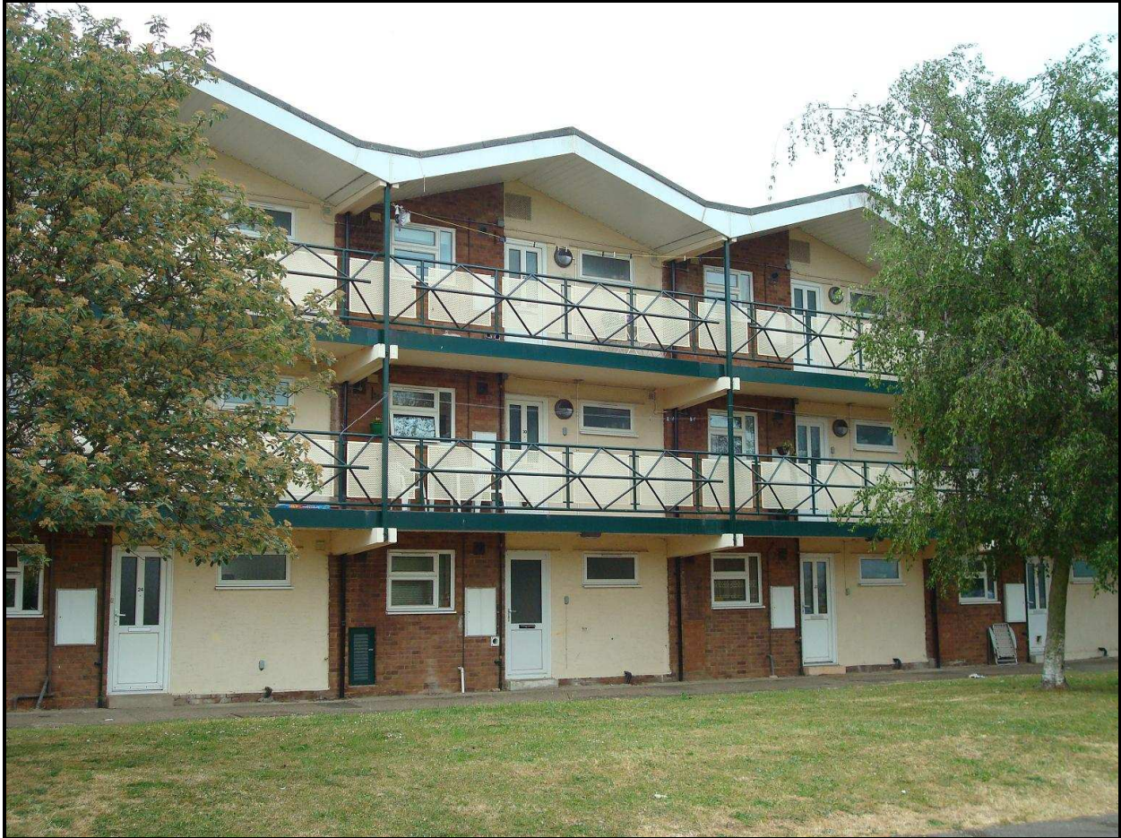
General view of block
